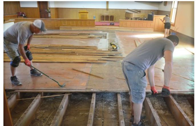
Work continues on new flooring in our sanctuary. The existing floor has been removed down to and including most of the original structure and later repair work. In respect for those who built the sanctuary for occupancy in 1870, a few boards that were still usable remain in the new floor. Coleman Home Repair Company is the contractor for the renovations.
