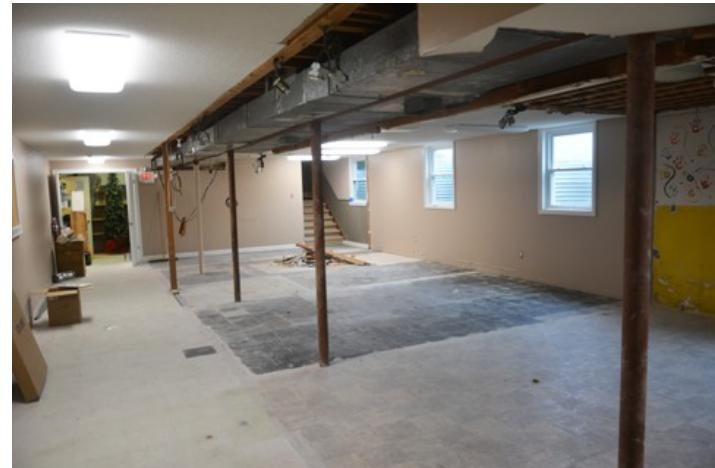
The new floor follows the original designed slope toward the front. The foundation was checked for needed repairs and upgrades, and a vapor barrier was placed on the ground. Work has begun on the altar area and alcove leading to fellowship hall.
